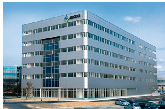
EIZO's new R&D center at its corporate headquarters in Hakusan, Japan
